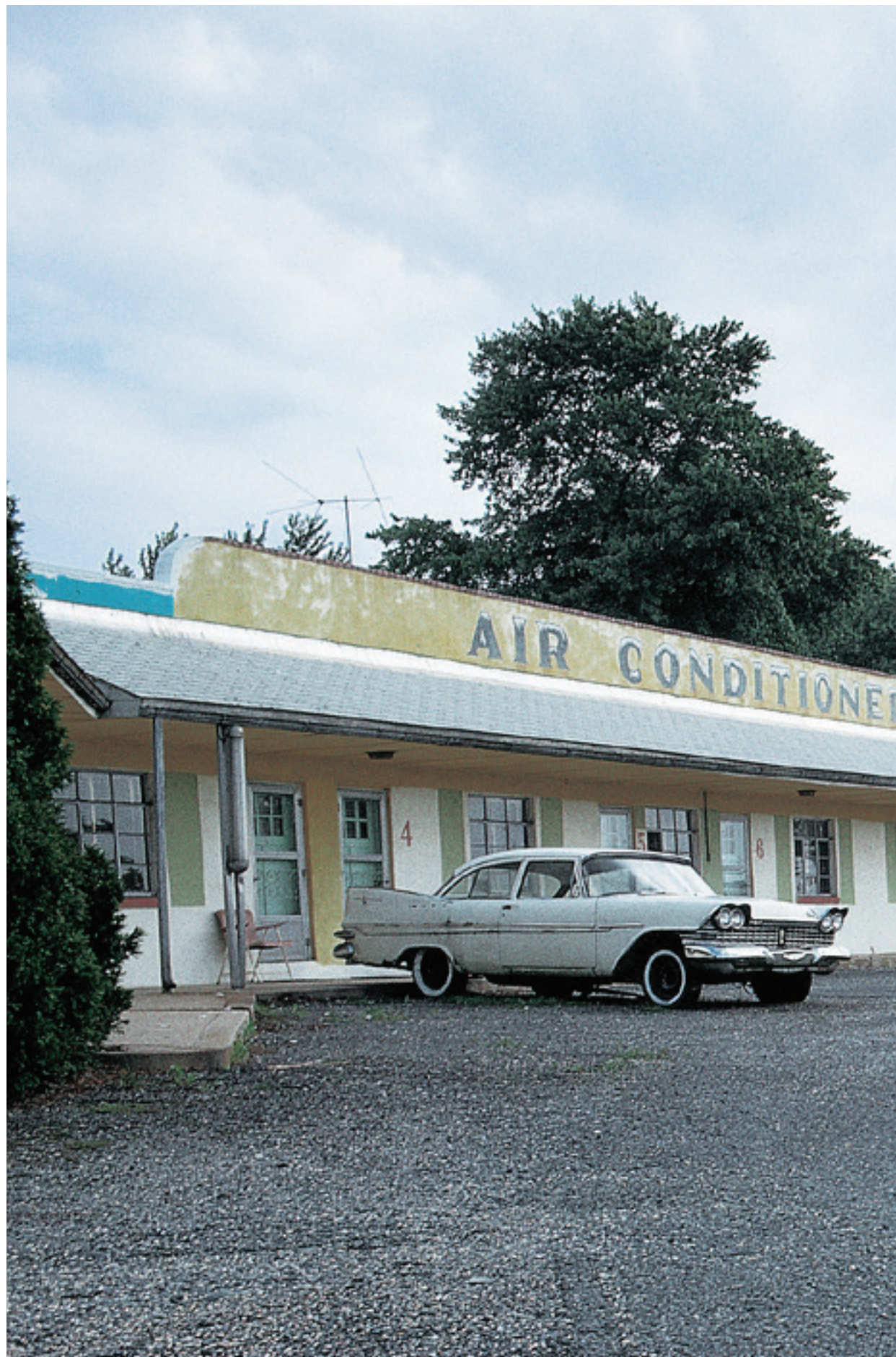
→ A motel on U.S. 40 north of Baltimore, Md. (seen here in July 1970), bears a typical single-story-row construction and boasts one of the luxuries of the post-World War II era: air conditioning.
